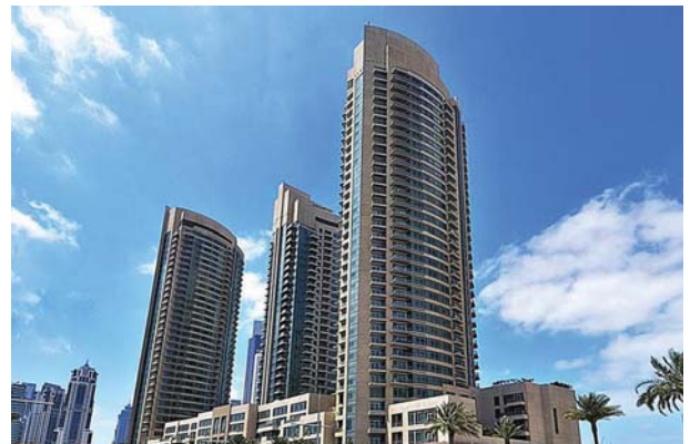
Burj Loft Project in Downtown, Dubai UAE
