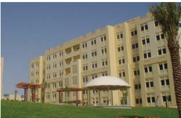
Adnoc Residential Complex at Khalidiya City, Abu Dhabi
